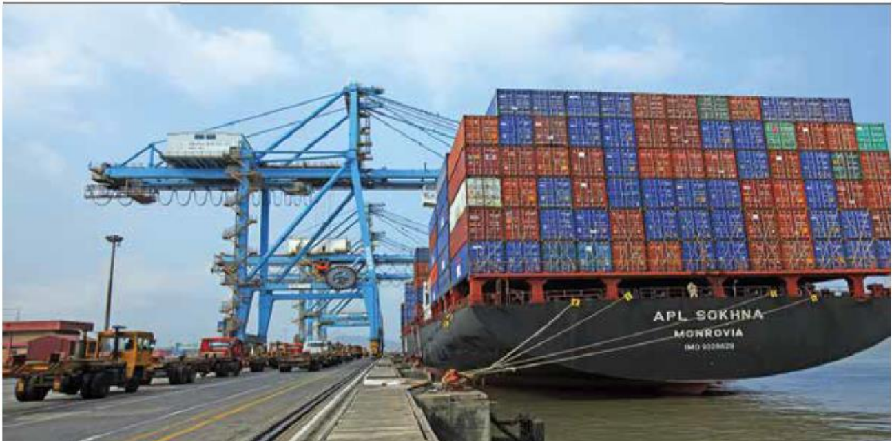
Figure 37: Jawaharlal Nehru Port Container Terminal 40
