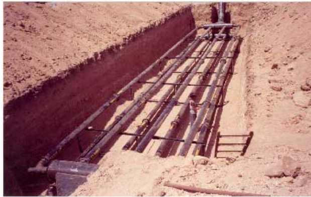
Fig 5. Earth tube heat exchanger before backfill
