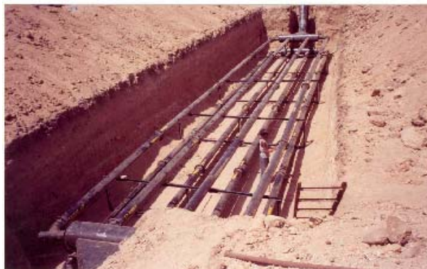
Fig. 4 (b). Earth tube heat exchanger before backfill
