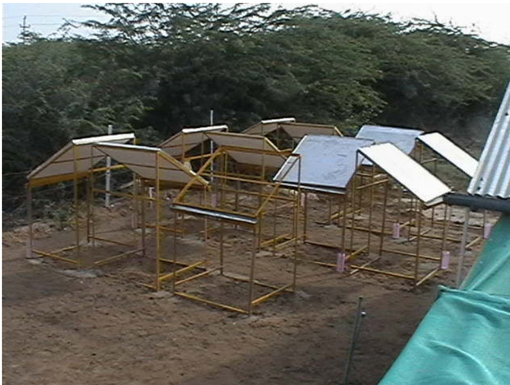
Figure 2. Condensers Test site at Kothara
